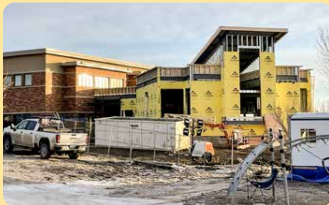
Bismarck Chapel construction, day 155.
