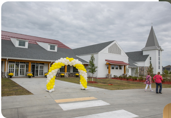
The completed Fargo expansion project houses the Gudrun R. Marx Chapel, Thrivent Mutual Funds Nutrition Center, and a gymnasium.
